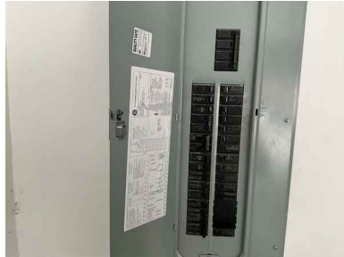
Main Service Panel Amperage: 200 Amp
