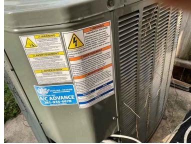
Approximate Condensing Unit BTU/Tonnage: 3 TON
